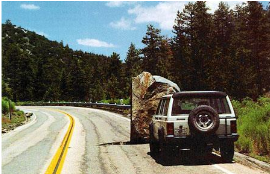
Highway 38 east of Barton Flats after the 1992 Big Bear Earthquake June 28, 1992
