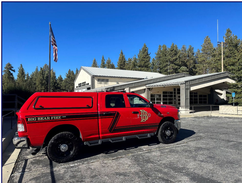
Figure 2: Big Bear Fire Department Headquarters
