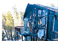
Residential Structure Fire in Big Bear
